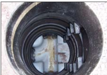
10.) Ready renovated manhole. Steps were removed on customer request
