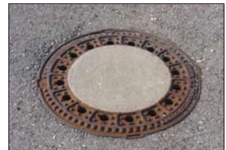
11.) Restoring of road construction incl. decoupled load cover
