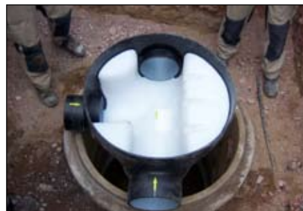
4.) Adapt the prefabricated channel with PE-socket
