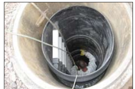
8.) Fitting the seals and chamber components - PE shaft system DN 800
