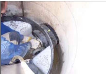
6.) Set the sealing plug to the in- and outlets, fill the gap with modified filling mortar
