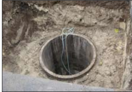
1.) Cut the asphalt, and lift the concrete cone
