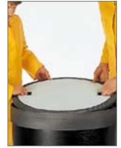
per end of the manhole ground or the manhole ring and must be checked for proper fitting. For manholes with diameters of DN 500 and DN 625 the transport security ring needs to be removed. Remove any burrs as well.
